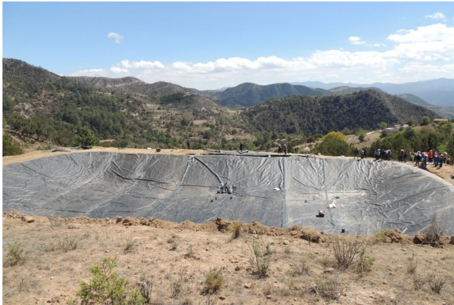
Photo 1: View of the Zacatepec Irrigation reservoir
