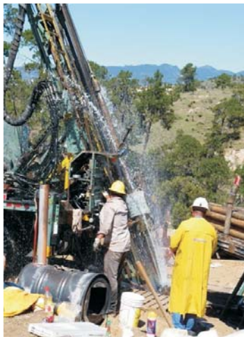
Drilling at the Tuligtic project Mexico
