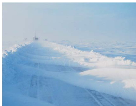
Winter Road on the ATW Project, N.W.T
